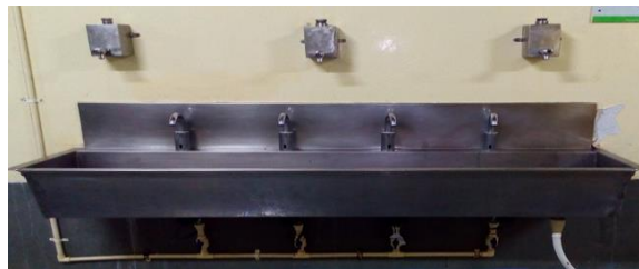
Figure 20: Foot Operated Hand Washing System
