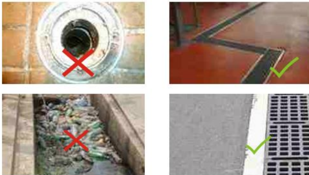
Figure7: Install covered drainage system inside the premises
